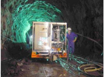
The technical solution proposed allows **EPC-France** to produce an explosive just at the end of the pumping hose. The explosive product (NITRAM TX1) is loaded into the borehole, as it is a low sensitivity explosive, it requires a powerful booster.
